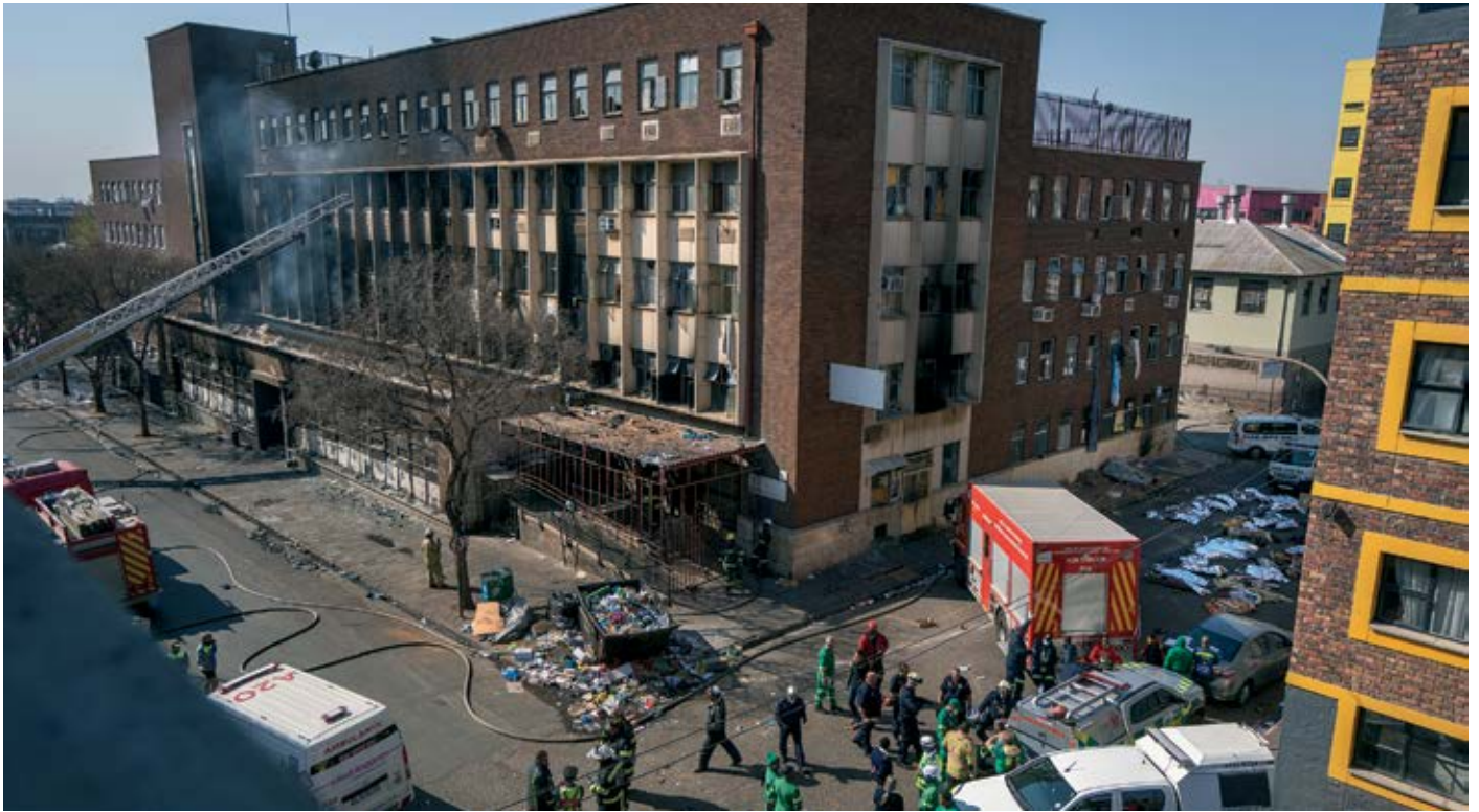
The building known as Usindiso Shelter after the deadly fire in August.
