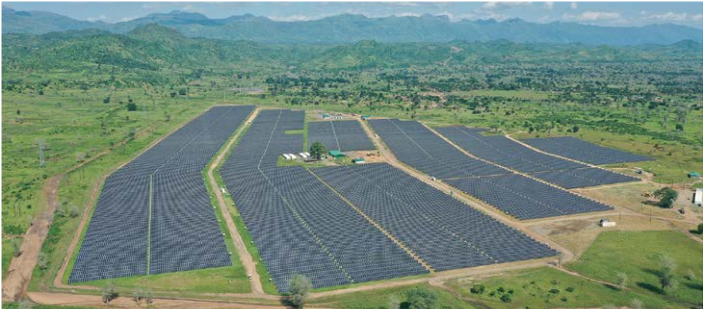
Golomoti is the first commercially operated solar-power plant in Malawi. It is a public-private partnership between Canadian independent power producer JCM Power, investment company InfraCo Africa, the Malawian government and the state-owned Electricity Supply Corporation of Malawi.
