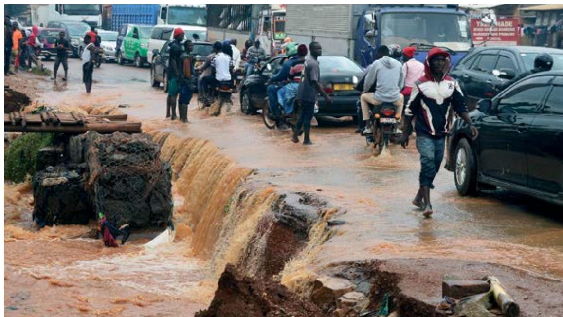
Kampala's streets after heavy rainfall.
