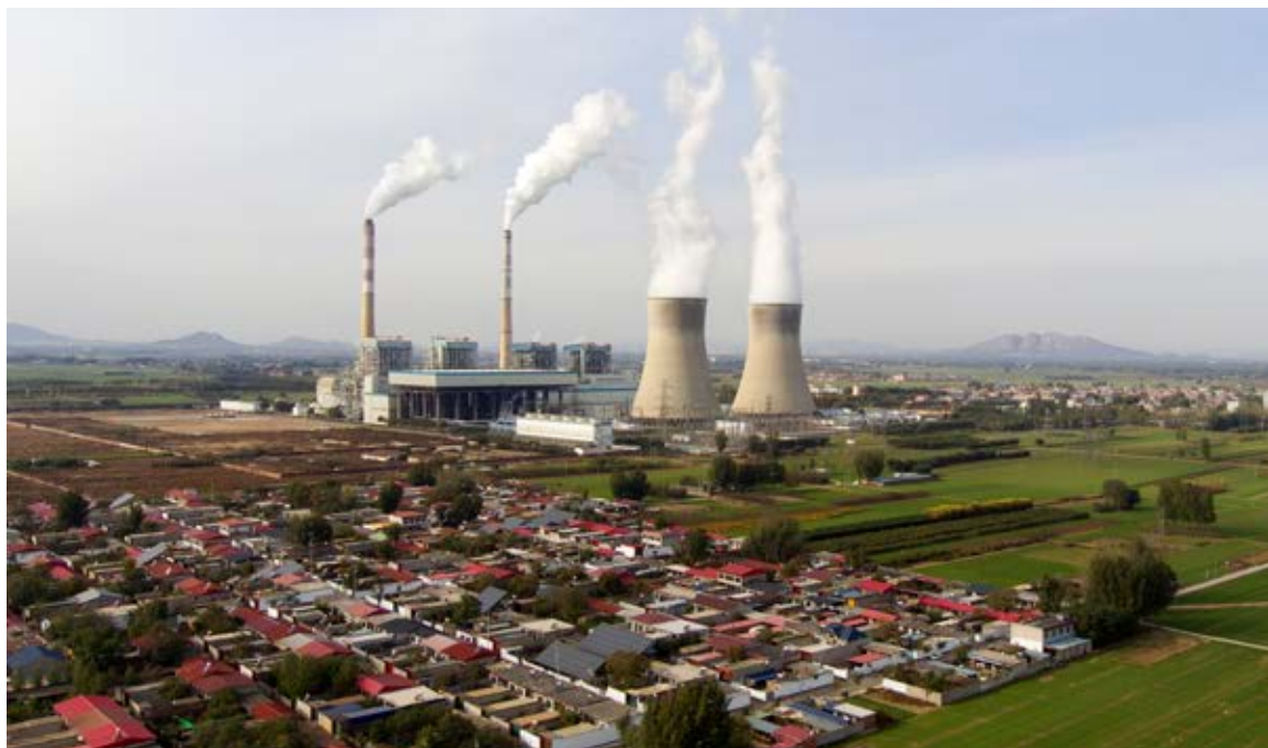
The Guohua coal-fired power plant in northern China.
