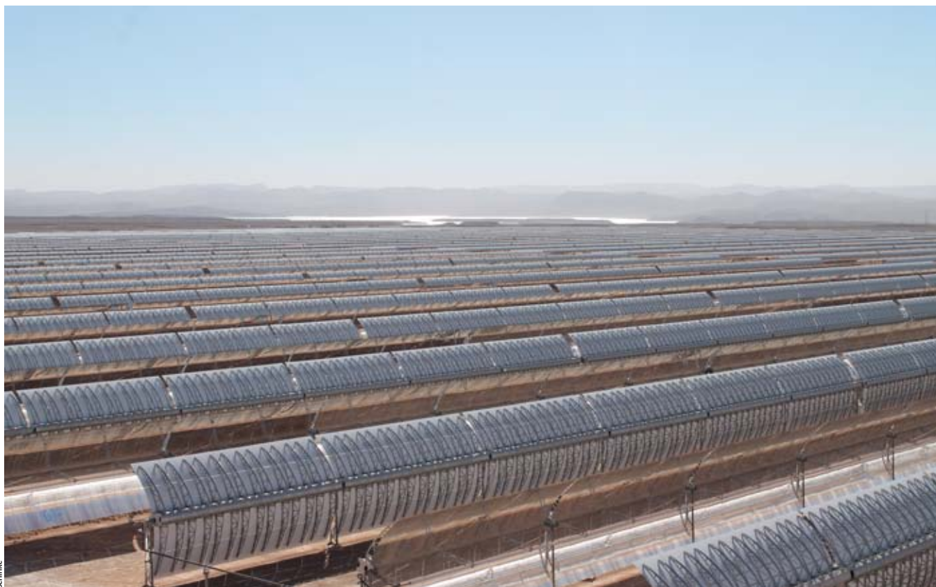
The concentrated solar power plant Noor I at the foot of the Atlas Mountains in Morocco.
