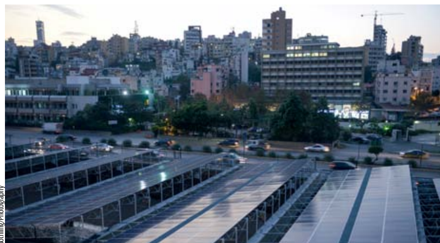
Renewable energy industries generate jobs worldwide. Solar panels on the Beirut River in Lebanon.
