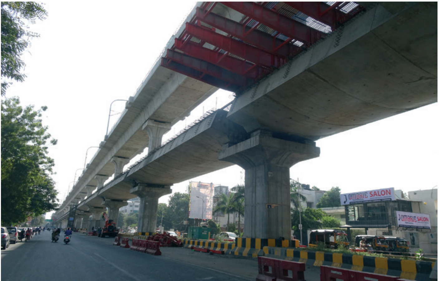
Maha Metro is particularly proud of the 4.5-kilometre-long double-decker section of the track that allows the metro to run above the street.
