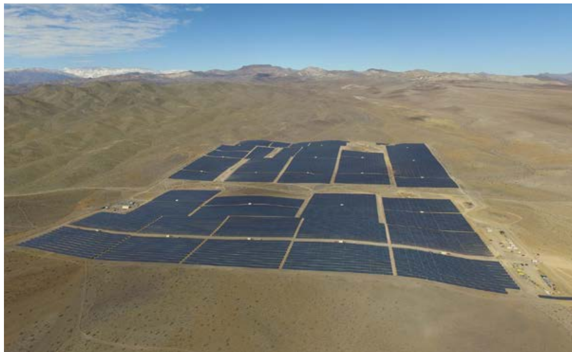
Solar panels installed in northern Chile.
