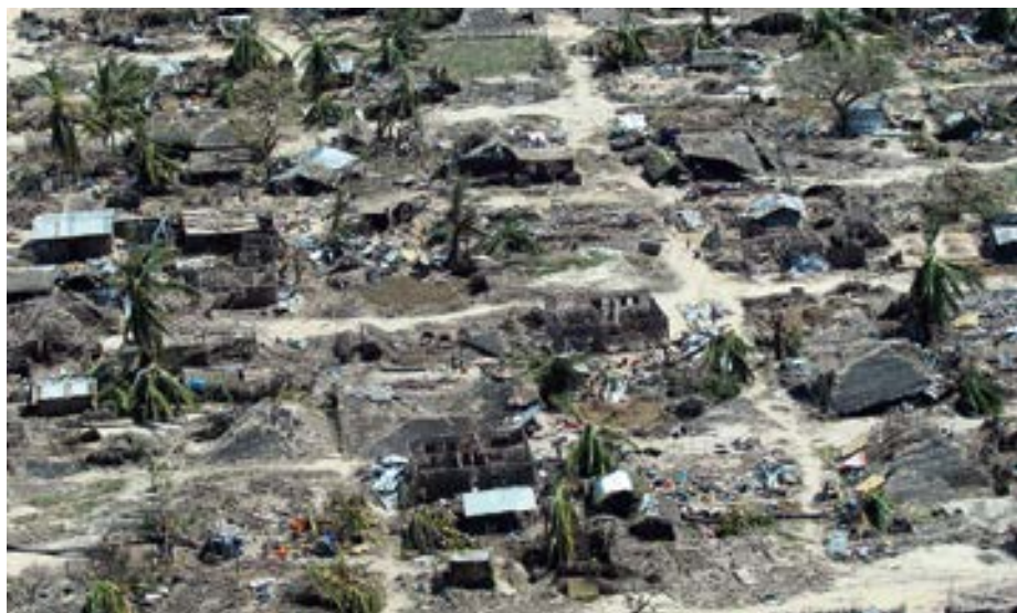
Cyclone damage on Ibo, a Mozambican island, in 2019.
