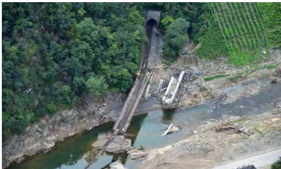
Flood damages in western Germany in August 2021.
