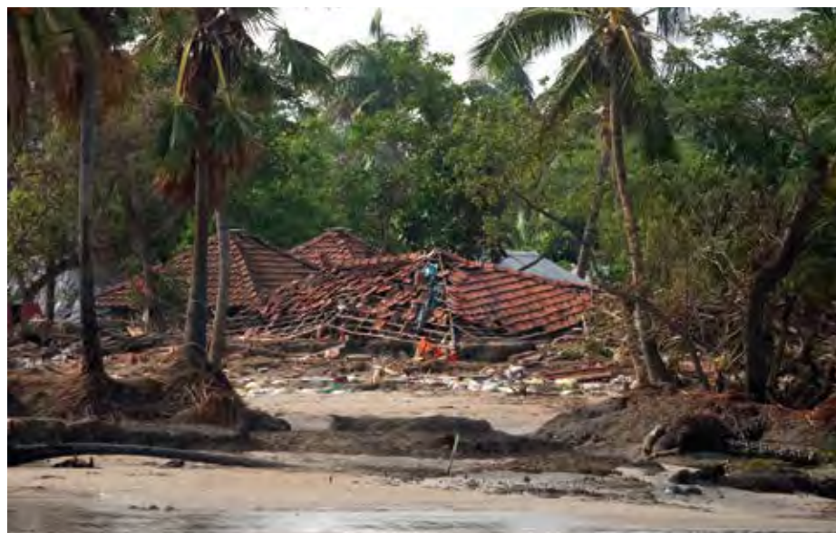
Poor communities suffer most: cyclone damage in West Bengal in May 2021.
