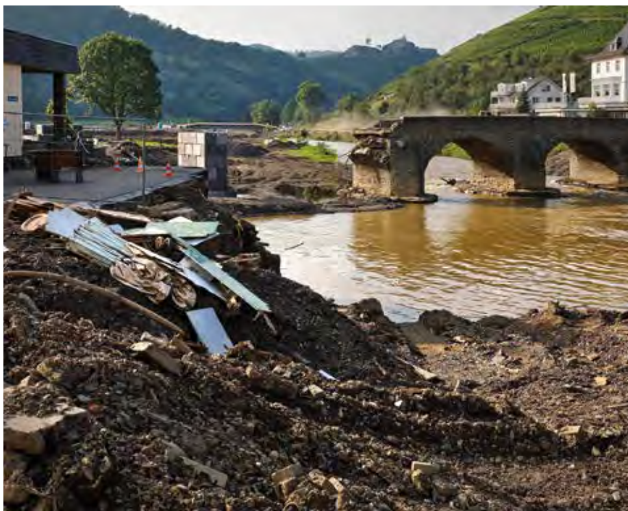
Devastating flood damage in Germany last summer.
